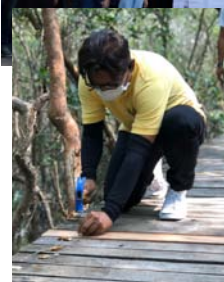
Corporate Social Responsibility activity by repaired bridge at Laem Phak Bia of the Royal Development Project
